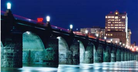
Figure 17 Lighting the arches of a bridge in Harrisburg, PA
