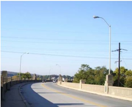
Figure 9 Existing "cobra head" light fixtures along bridge
