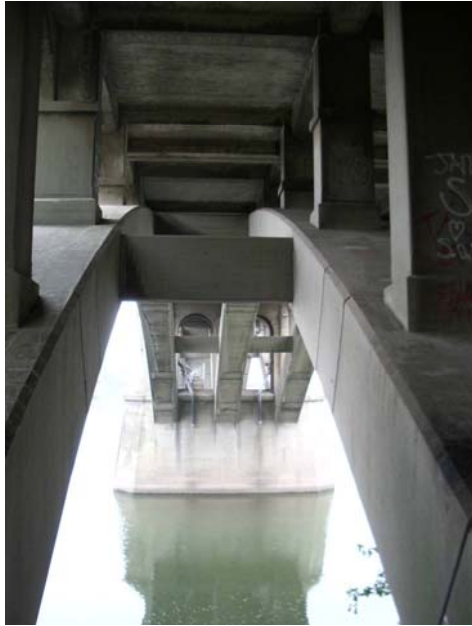
Figure 24 Underside of bridge is accessible from the shore
