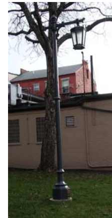
Figure 7 Six-sided lantern fixture and pole, at Columbia Historic Preservation Society
